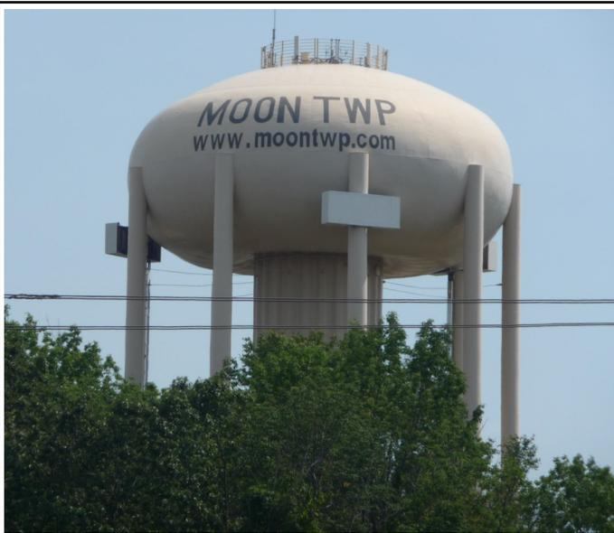
A Pennsylvania water utility compared the chlorine reading of their PHi mixed water tank to their two other non-mixed tanks. They discovered that the mixed tank had a free chlorine reading of .3 ppm in and .2 ppm out. The non-mixed tanks had a free CL reading of .8 ppm in and .03 ppm out and 1.1 ppm in and .15 out, respectively.
