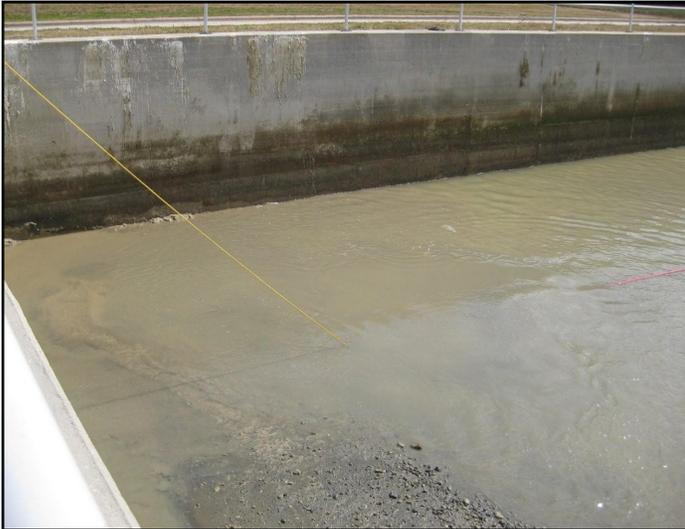
The key to effective drinking water filtration is regular backwashing of the filters, and as long as mud remains in thin suspension in a backwash holding basin, it can be pumped out.
