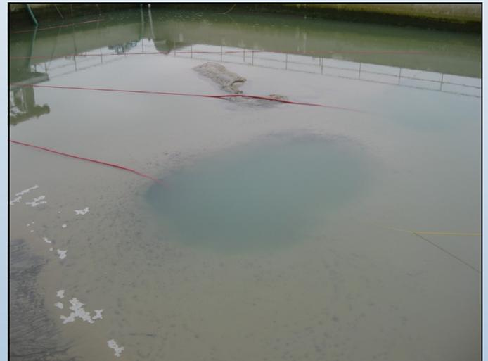
After a short period of mixing, a zone is cleared of mud, and the forming plate is moved to a new zone.
