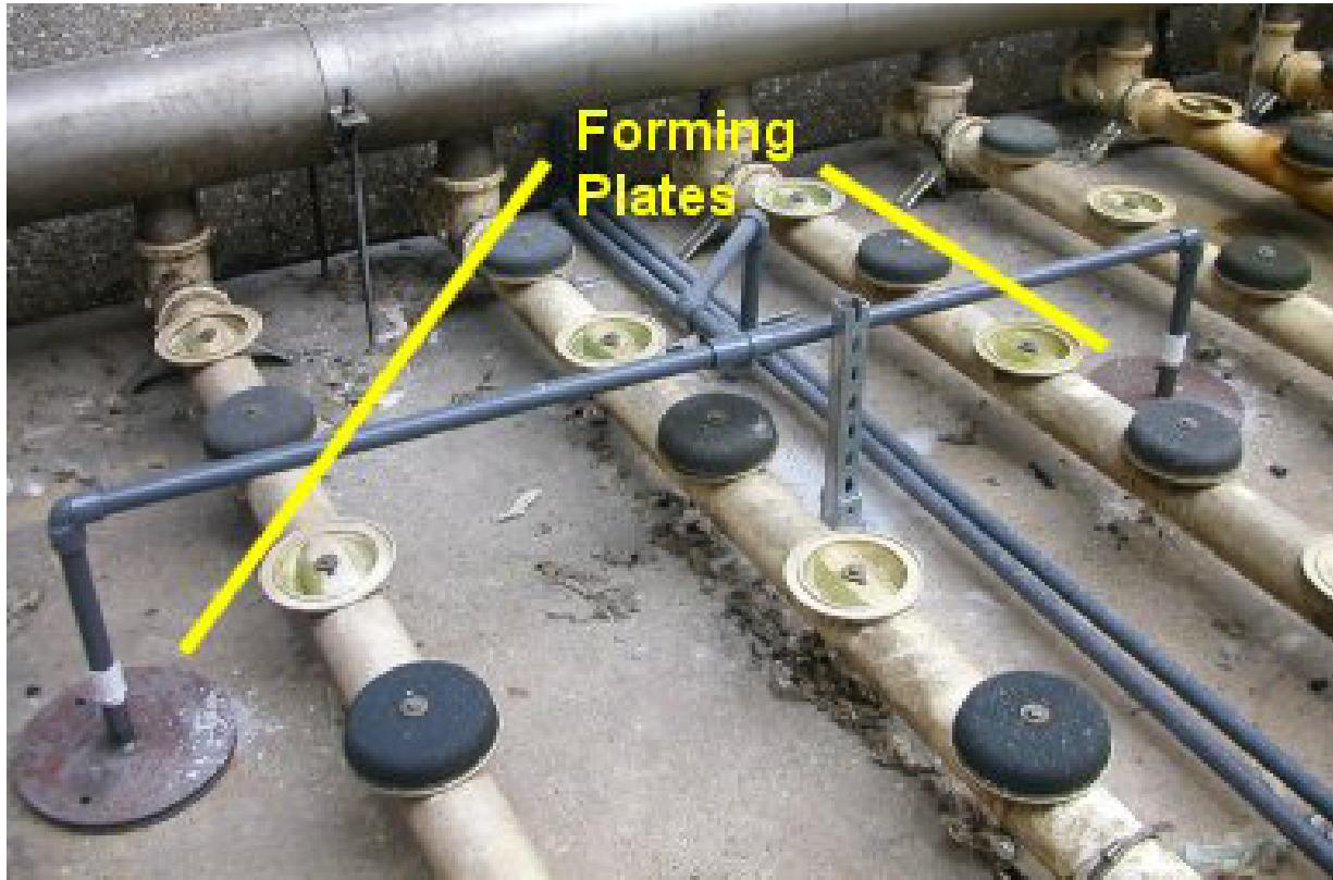
**Figure 1. Hydro-Pulse bubble forming plates at the bottom of tank**
