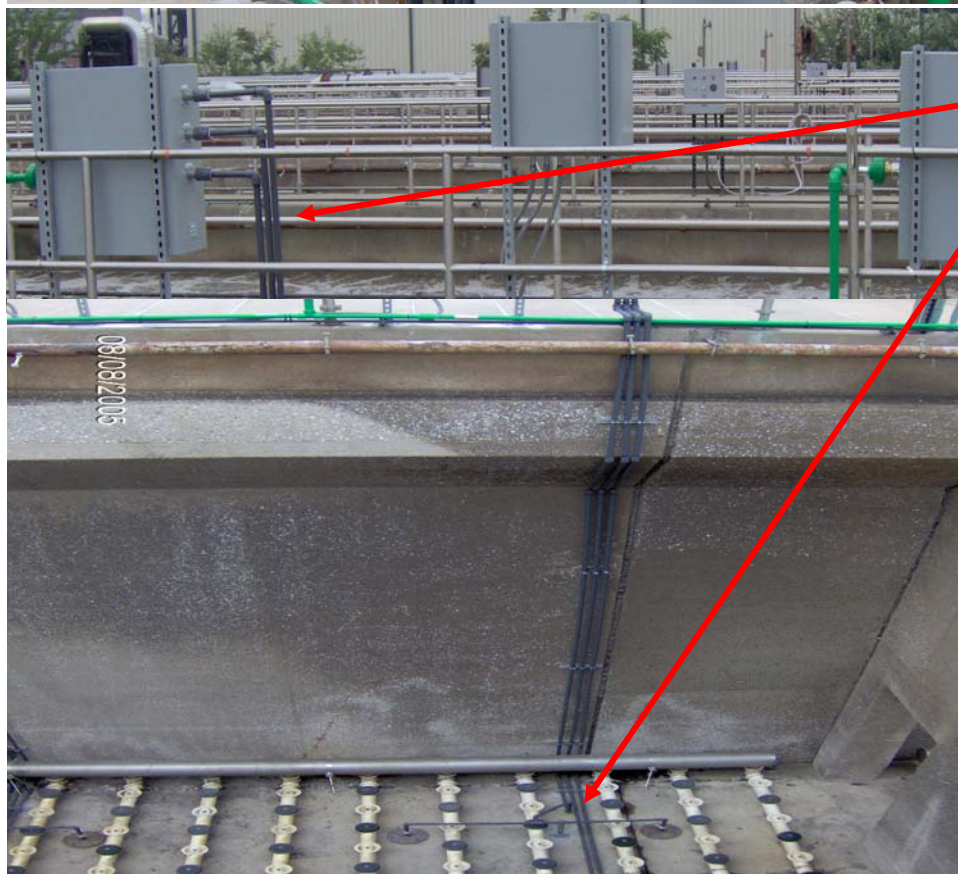
Figure 9. Air Piping layout photographs at the Red Hook WPCP for the PHI 9/18 Mixing System
