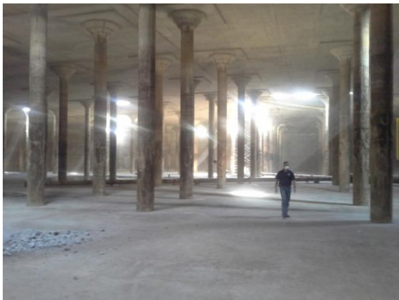
View: Inside Reservoir
